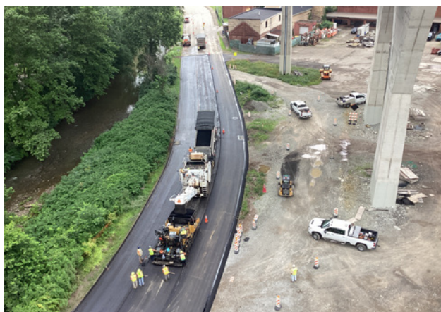
Asphalt paving on Peters Creek Road.
