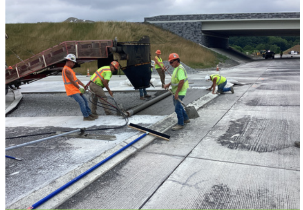
Mountable curb concrete placement at Jefferson Boulevard.
