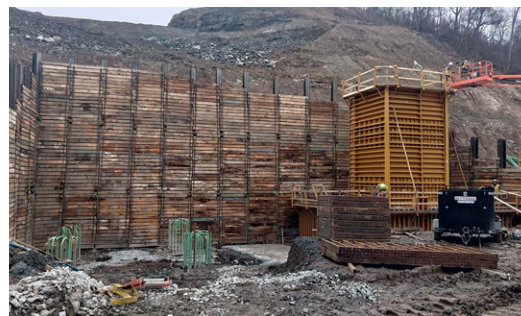
Pier construction for bridges over Coal Valley Road.
