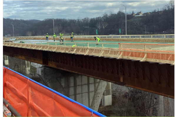
Deck reinforcement bar installation for bridge over SR 51.
