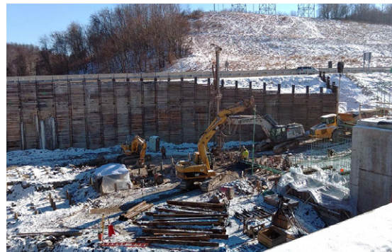
Abutment work for bridges over S.R. 51.
