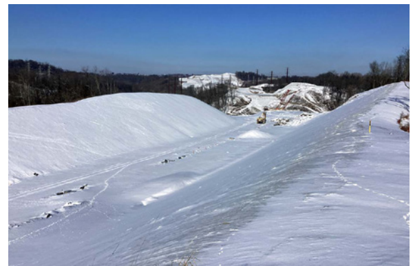
New highway alignment looking north across New England Road.
