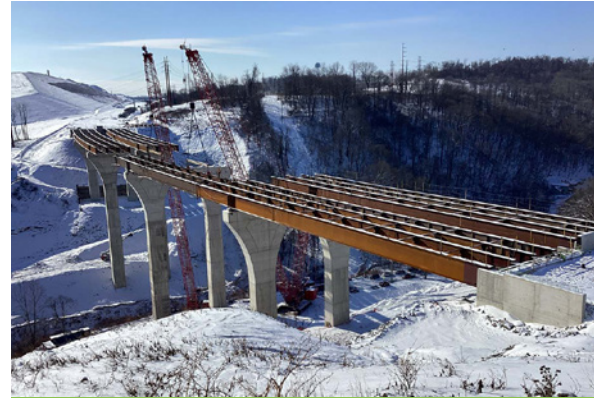
Construction progress bridges over Coal Valley Road.
