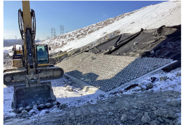
Articulating cellular block slope wall construction.
