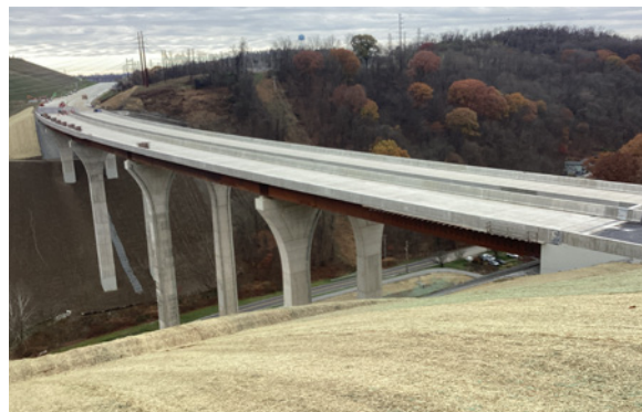
Bridges over Coal Valley Road.
