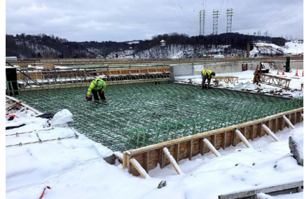
Approach slab rebar tying for bridge over SR 51.
