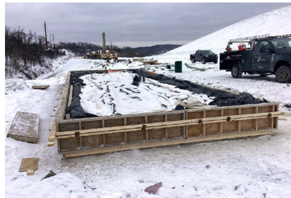
Toll building foundation construction.
