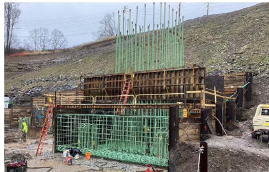
Construction of the Pier 2 footing for the bridge over Coal Valley Road.
