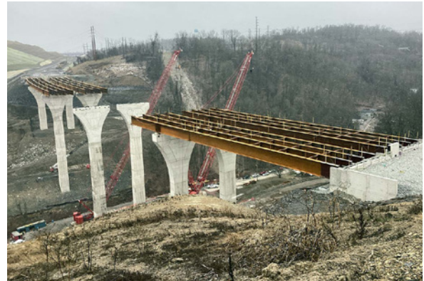
Construction progress bridges over Coal Valley Road.
