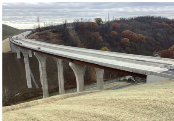
Bridges over Coal Valley Road.
