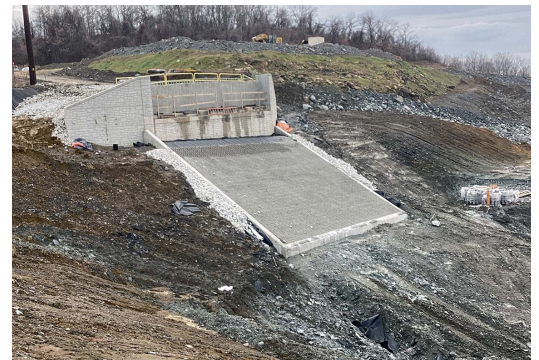
MF 403 Abut 1 Articulating Block Slope Wall (Future Bridge Carrying SR885 Over New Highway).
