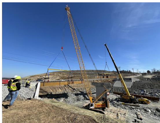
Steel girder erection for future SR 885 bridge over new highway.
