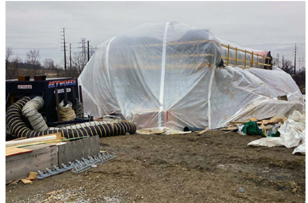
Heaters help the concrete cure for the electronic tolling building.
