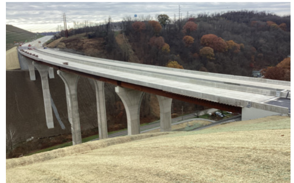
Bridges over Coal Valley Road.
