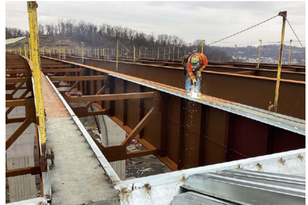
Welding on bridge over Coal Valley Road.
