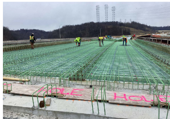
Reinforcement bar installation for bridge over SR51.
