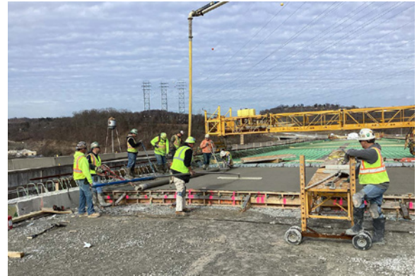
Approach slab construction for bridge over SR51.
