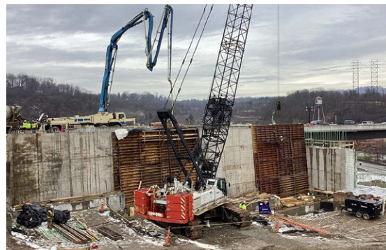
Concrete placement for bridges over S.R. 51.
