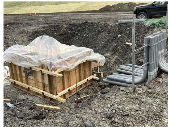
Toll gantry precast column footing.
