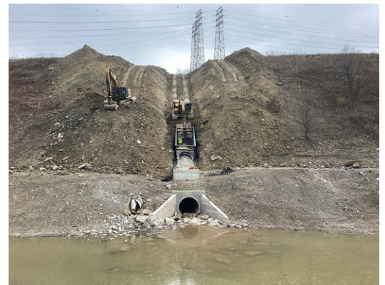
Installation of a 60 inch reinforced concrete pipe culvert
