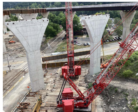
Steel girder erection for bridges over SR 51.
