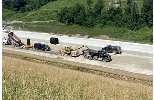
Pavement base drain installation for new highway at toll location.
