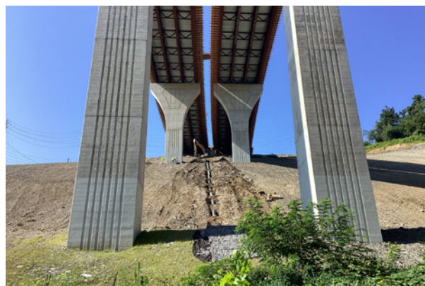
Scupper drain installation for Coal Valley Road bridges.
