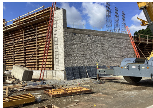
Adding the architectural design treatment to the bridge over S.R. 51
