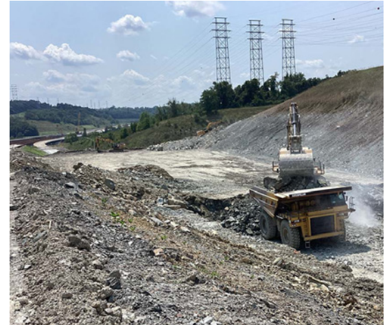
Bulk excavation near Jefferson Boulevard.
