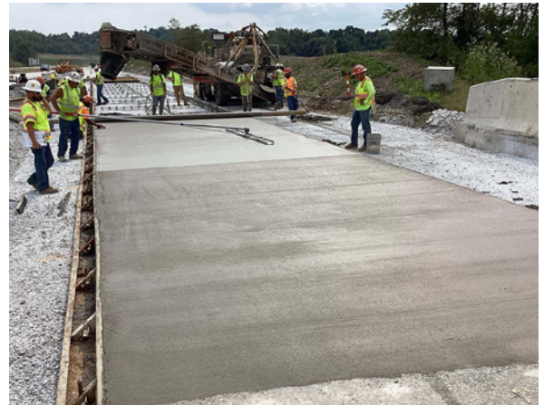
Bridge transition concrete paving
