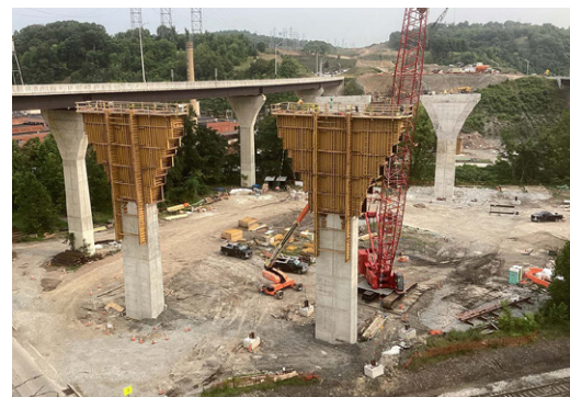
Work continues on the bridge piers over SR 51.
