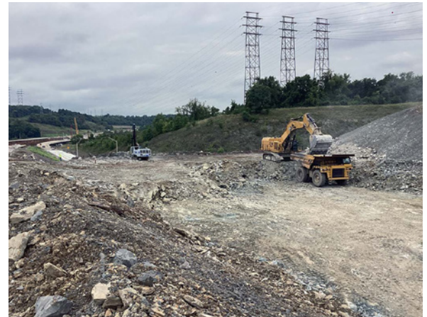
Bulk excavation near Jefferson Boulevard.
