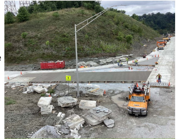
Long-life concrete paving PTC-43 southbound off ramp to Jefferson Boulevard.
