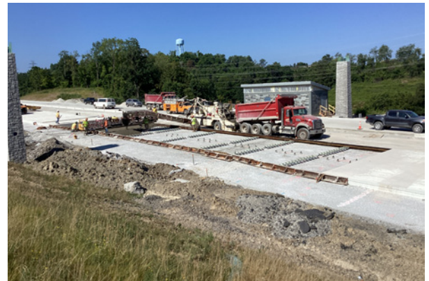
Concrete roadway placement through tolling location.
