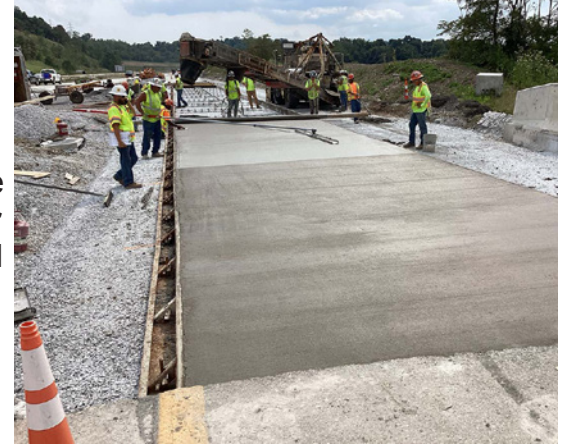
Bridge transition concrete paving.
