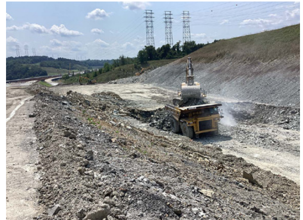
Bulk excavation near Jefferson Boulevard.
