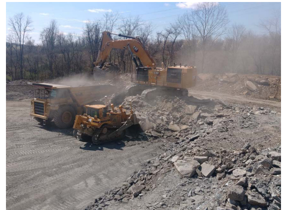
Bulk excavation for new highway.
