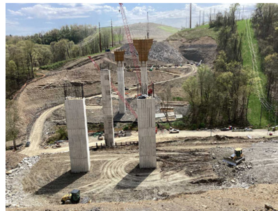
Bridges over Coal Valley Road construction progress.
