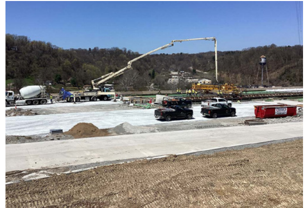
Concrete pump truck used for deck placement over SR 51.
