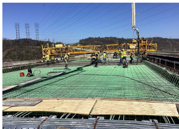
Concrete deck placement for bridge over SR 51.
