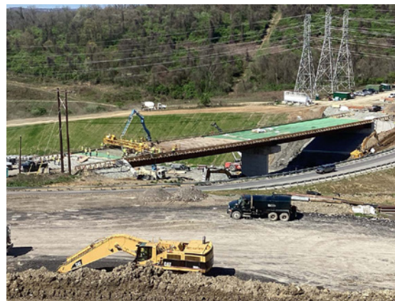
Concrete deck placement for new SR 885 bridge.
