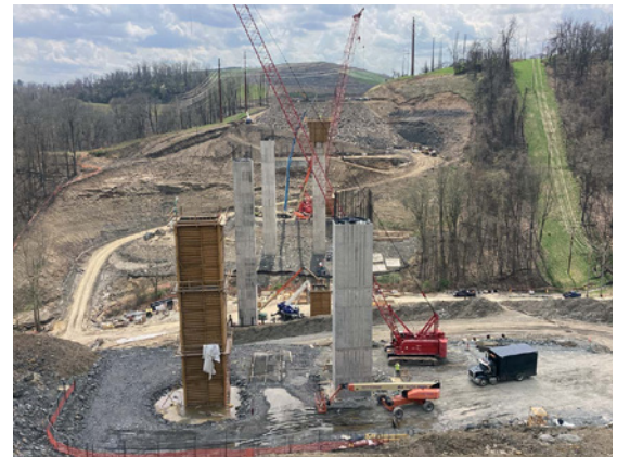
Bridges over Coal Valley Road construction progress
