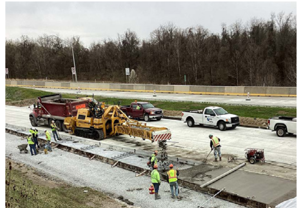
Concrete paving for Jefferson Boulevard northbound off ramp.
