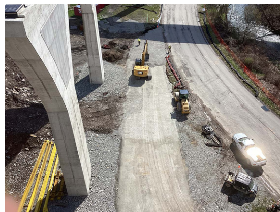
Peters Creek Road temporary runaround for beam erection.
