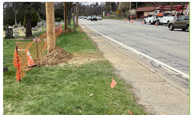
Temporary traffic signal work in Dravosburg.
