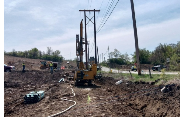
Drilling for Mine Grouting along SR 885.
