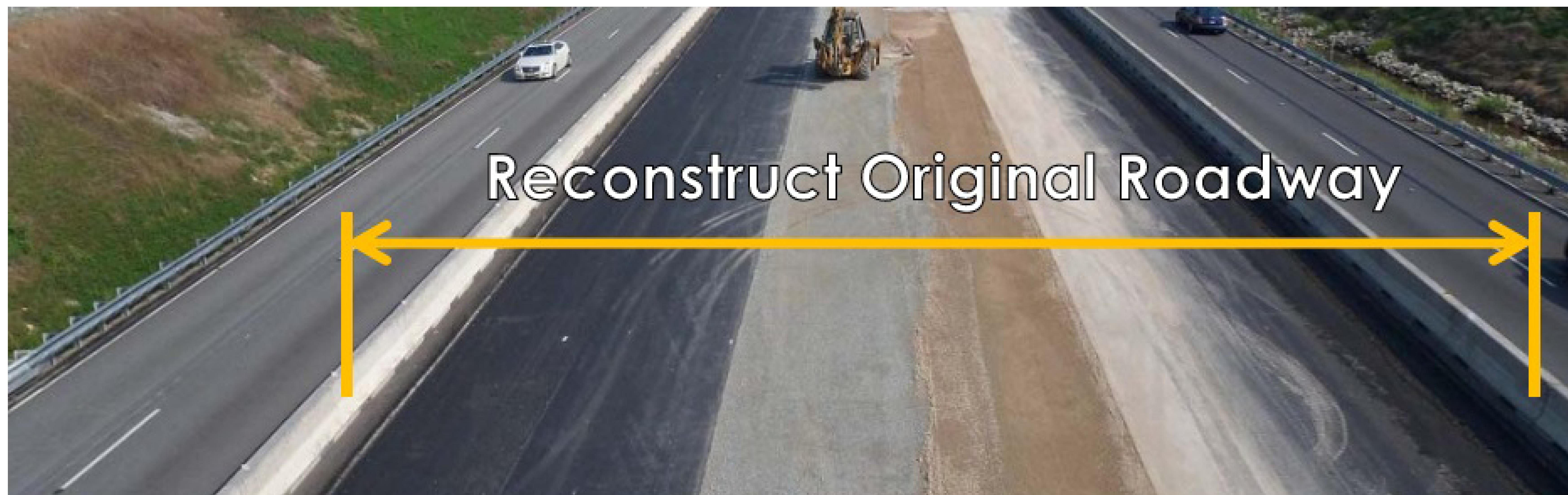
Second Major Construction Stage
