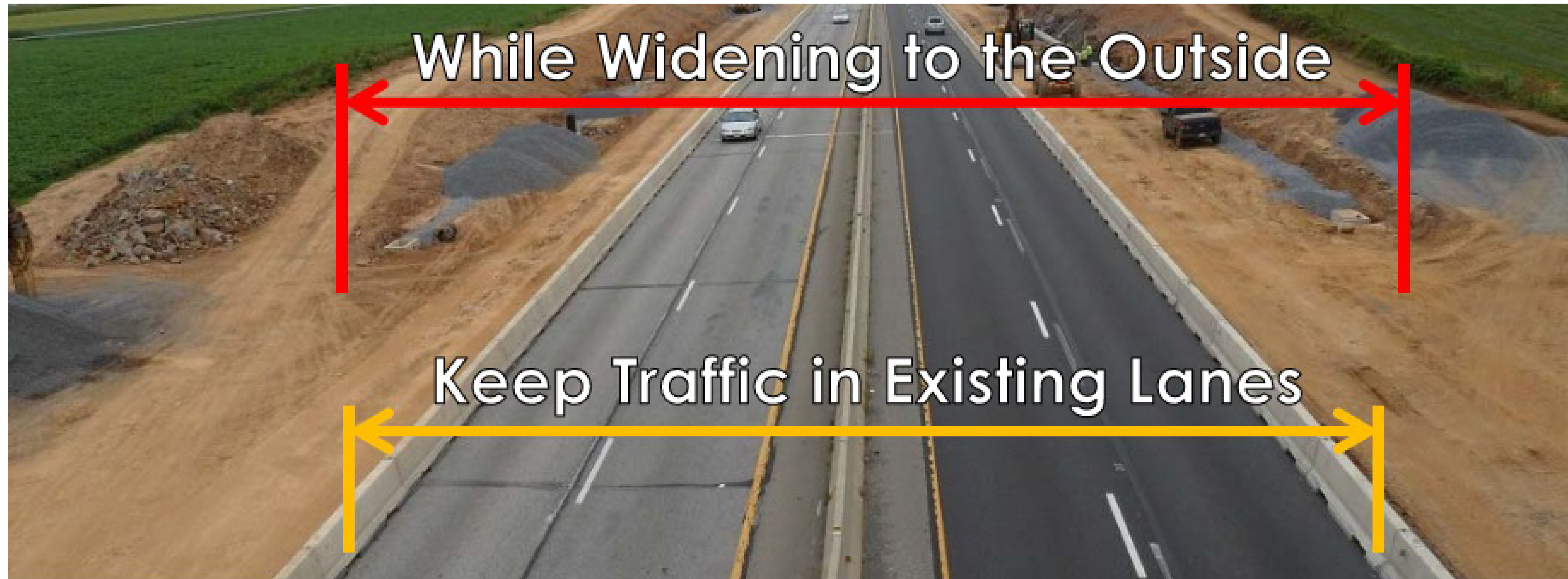
First Major Construction Stage
