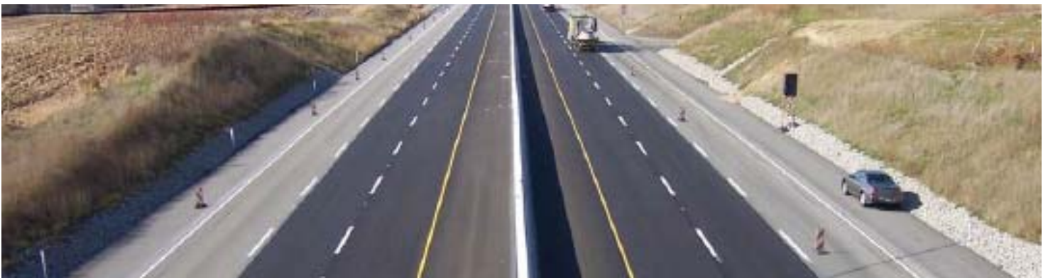
← Typical Total Reconstruction Section 122' out-to-out →
