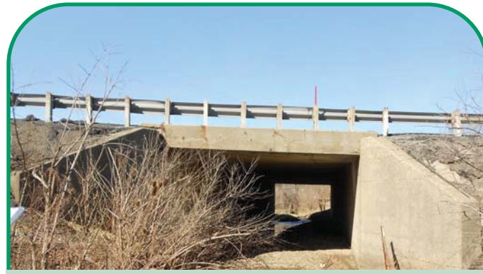
Existing WB-401 Bridge over Tributary of Brush Creek
