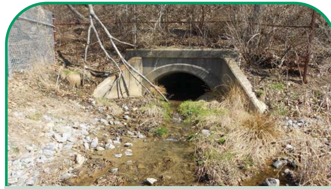
Existing WB-403B Culvert conveying Tributary of Brush Creek
