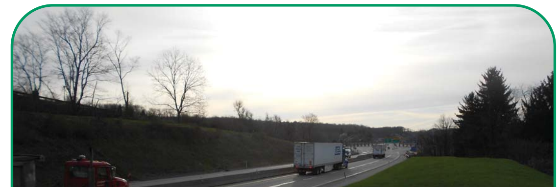
Milepost 30.5 — Looking eastbound.
