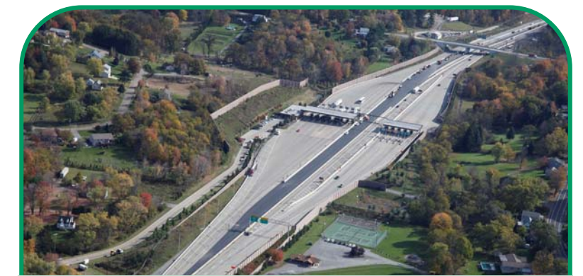
Warrendale Toll Plaza looking eastbound.
