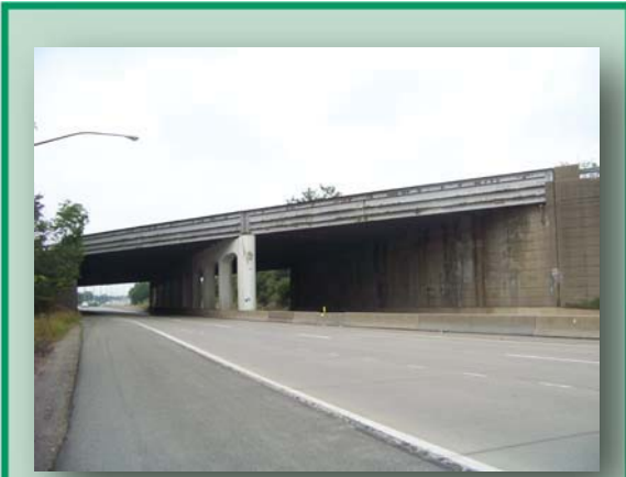
Replacement of Mainline Bridge (WB-402) over SR 0019 (Perry Highway) at Milepost 29.70
