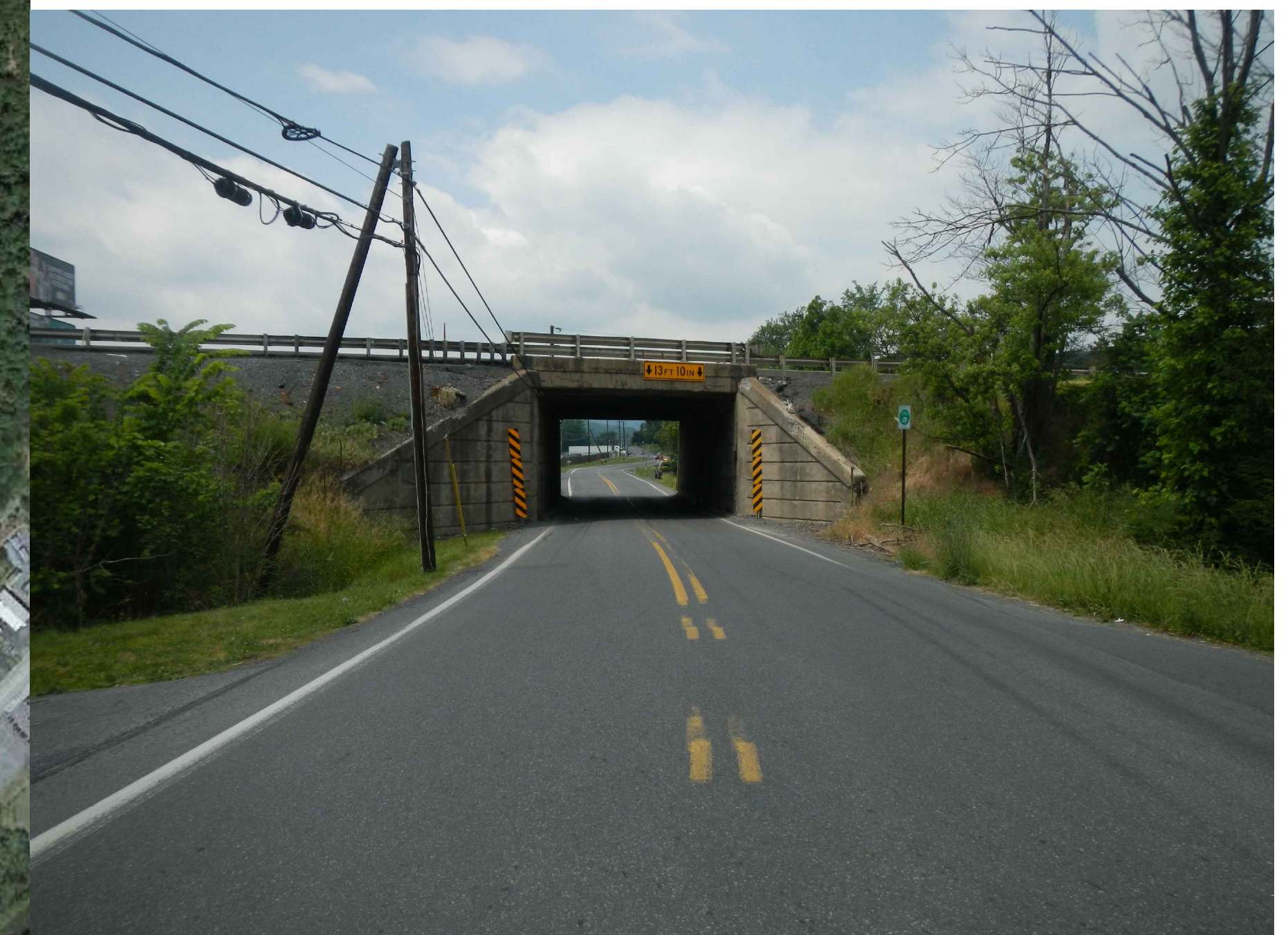
S.R. 1001 (SUNNYSIDE ROAD) LOOKING SOUTHWEST AT B-140
