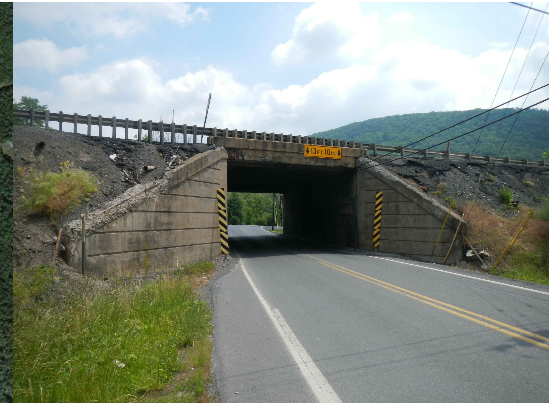
S.R. 1001 (SUNNYSIDE ROAD) LOOKING NORTHEAST AT B-140
