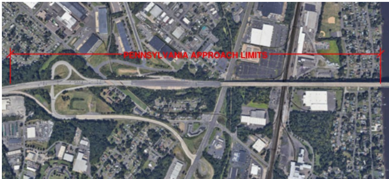
Figure IV.1 – Aerial View of the Pennsylvania Approach (2022)
