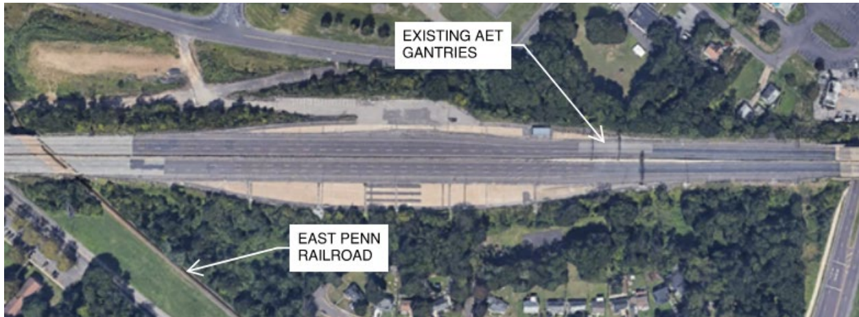
Figure IV.3 – Aerial View of Former Mainline Toll Plaza Area (2022)
