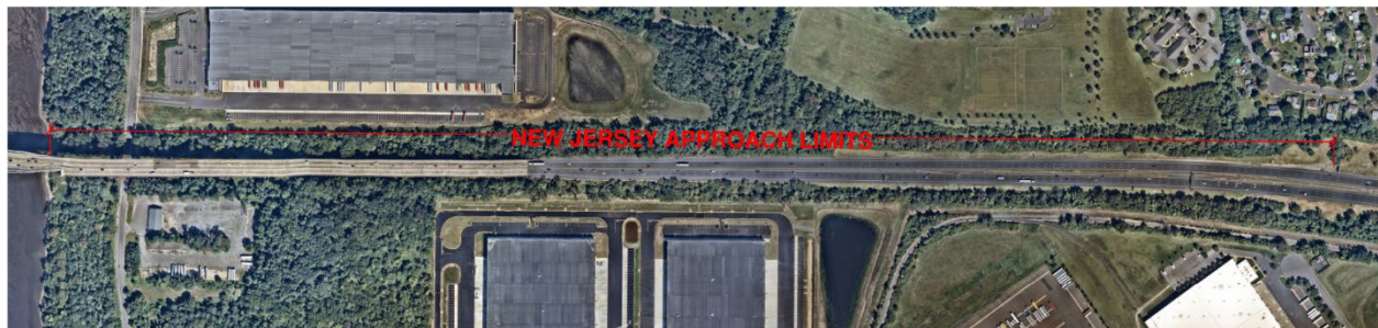
Figure IV.8 – Aerial View of the New Jersey Approach (2022)
