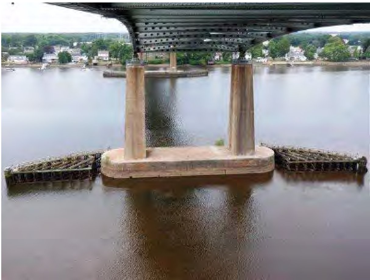
Photo 10: Pier 19, looking west (Photo: ATANE Consulting, 2022)
