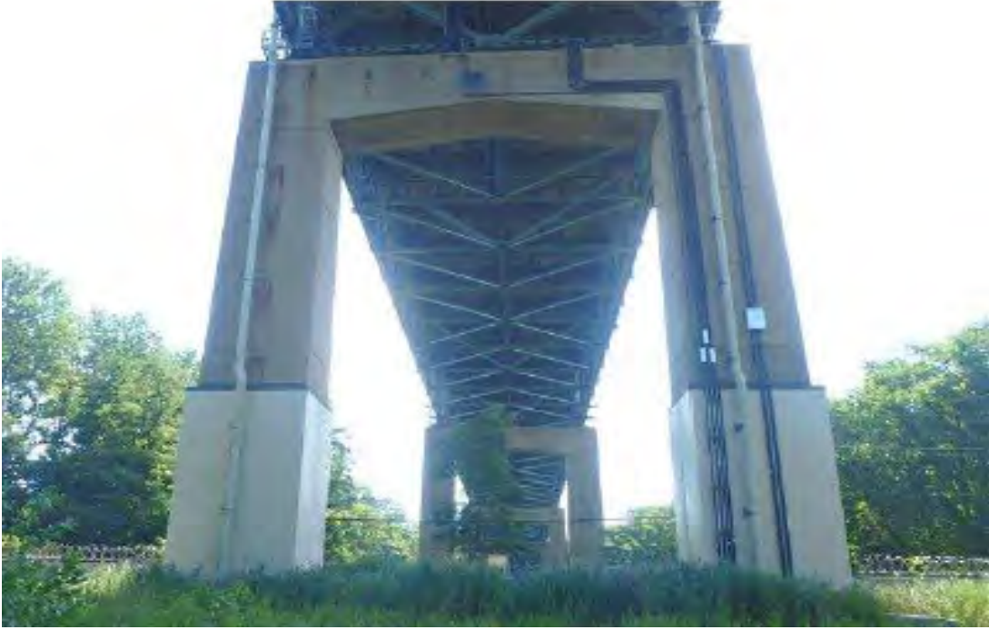
Photo 11: Pier 21, looking east (Photo: ATANE Consulting, 2022)
