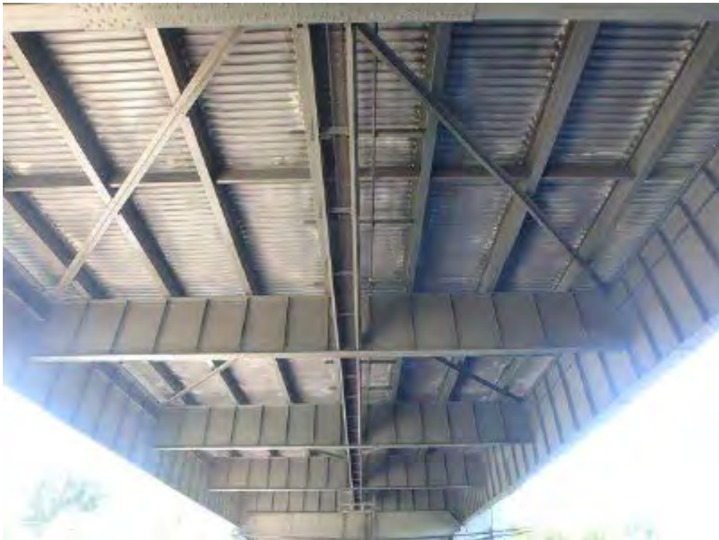
Photo 6: Steel Girder/Floorbeam/Stringer spans, looking west (Photo: ATANE Consulting, 2022)
