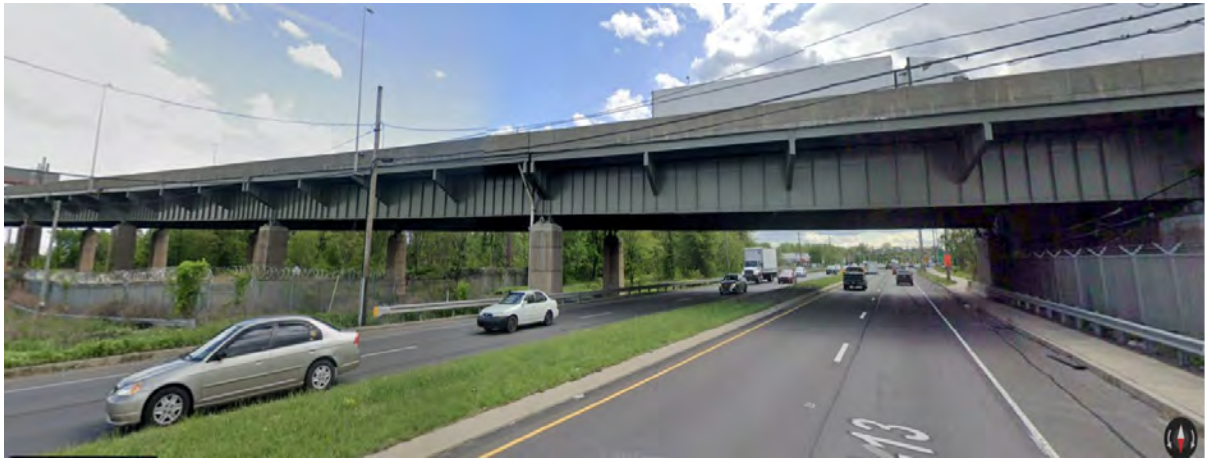
Photo 9: Girder/Floorbeam/Stringer spans, Pennsylvania side, looking north (Photo: Google Streetview, 2023)
