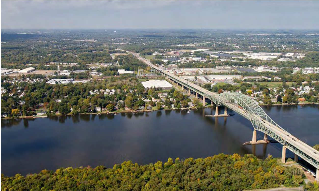
Figure 1-2 Bridge View Looking Northwest (Looking Towards Pennsylvania)
