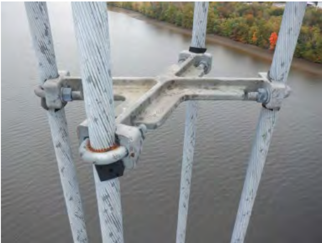
Photo 12: Replaced Suspender, looking north (ATANE Consulting, 2022)
