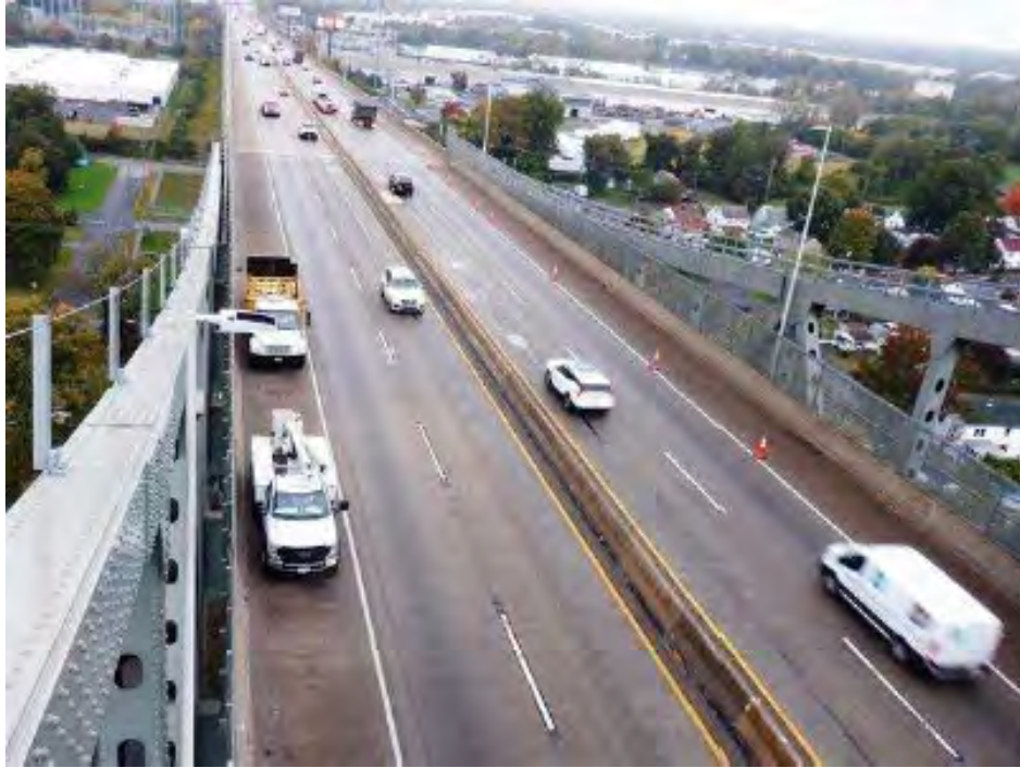
Photo 3: Top of Deck (Spans 1 to 18 shown), looking west (Photo: ATANE Consulting, 2022)
