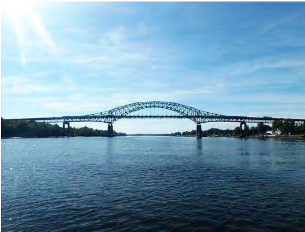
Photo 2: North elevation, Spans 18 to 20, looking south (Photo: ATANE Consulting, 2022)
