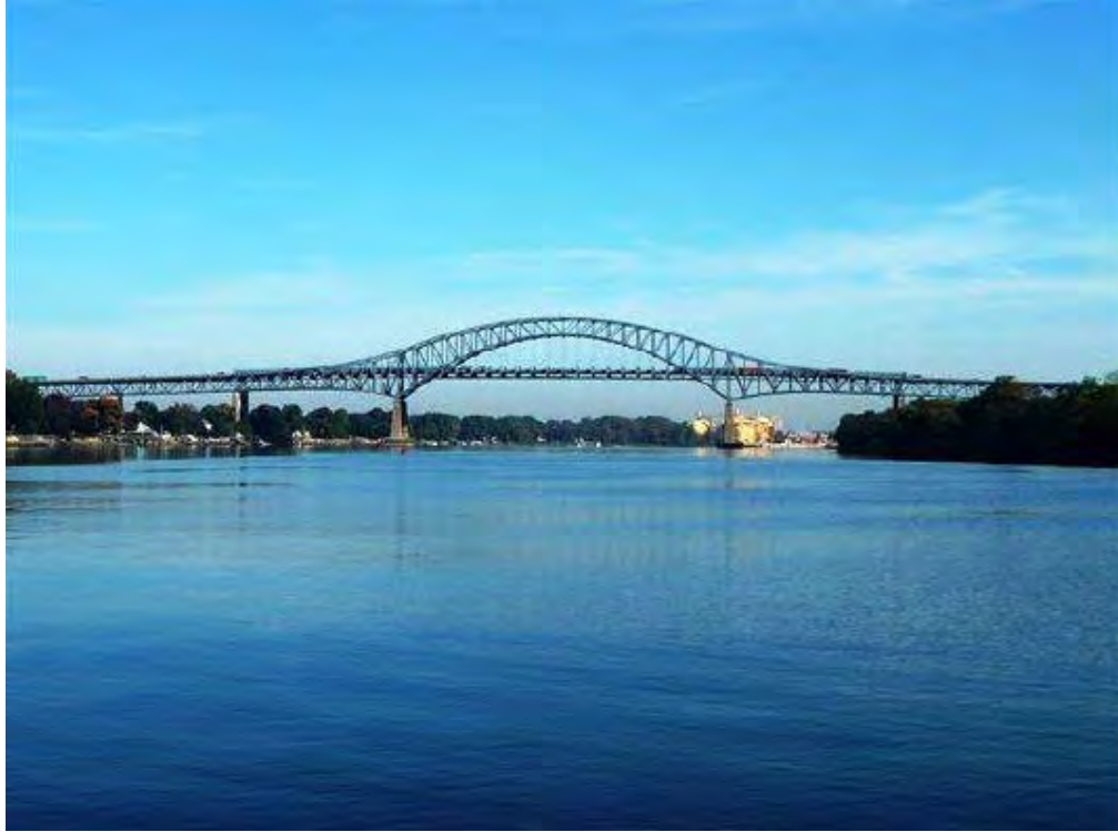
Photo 1: South elevation, Spans 18 to 20, looking north (Photo: ATANE Consulting, 2022)
