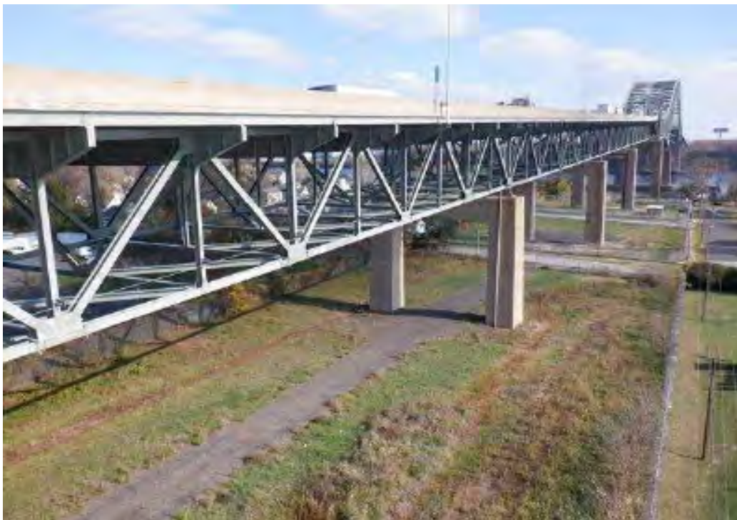
Photo 8: Deck truss approach spans, Pennsylvania side, looking northeast (Photo: ATANE Consulting, 2022)
