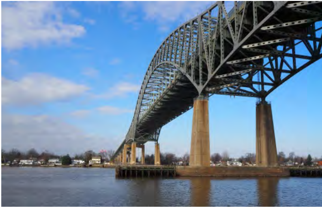
Photo 7: Main spans, looking west from New Jersey (Photo: HDR, 2024)
