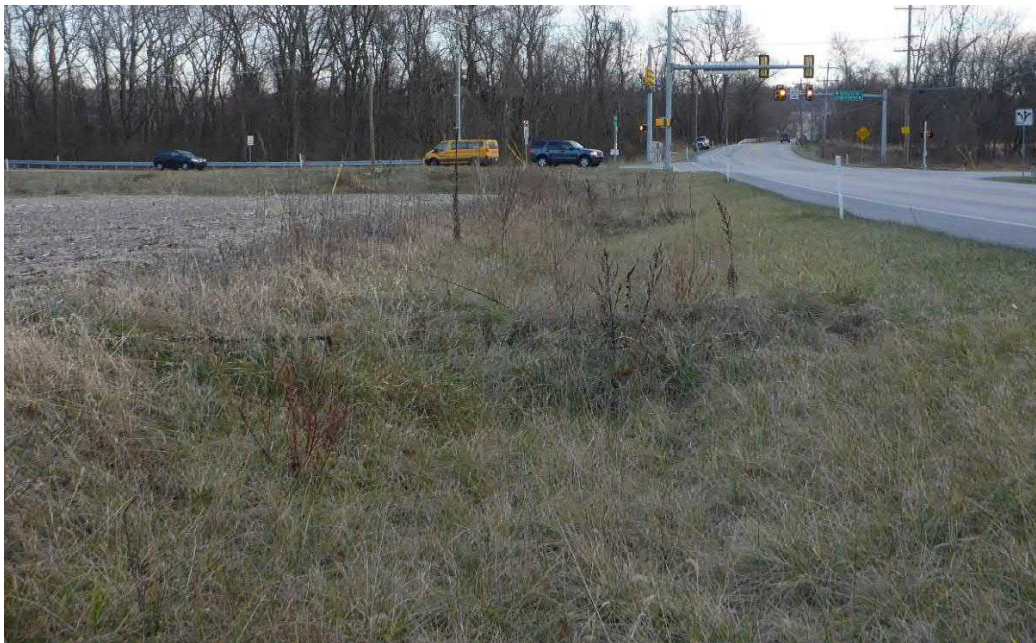
Figure 6.11.2: Vegetated Swale with Check Dams (VSC) (photo c/o: PennDOT)
