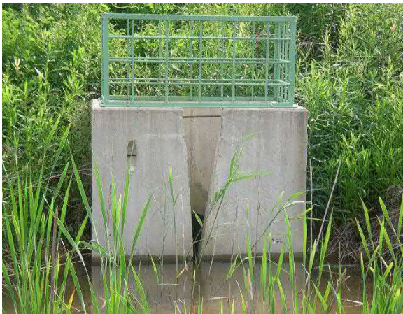
V-notch weir with top mounted trash rack
