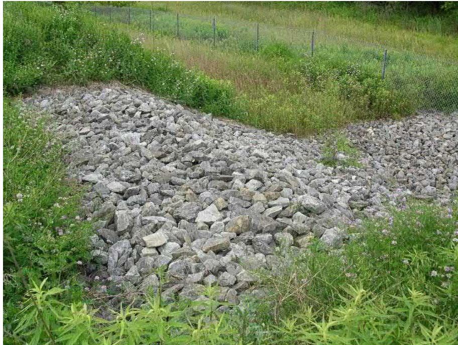
Figure 5.10.1: Emergency Spillway (photo c/o: PennDOT)
