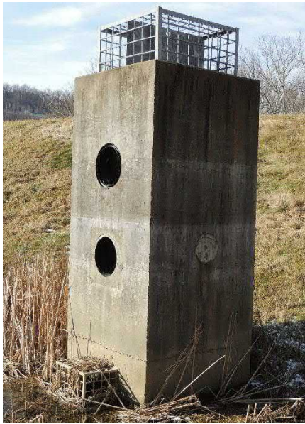
Circular orifices with trash rack on low flow orifice and top (photos c/o: PTC)
