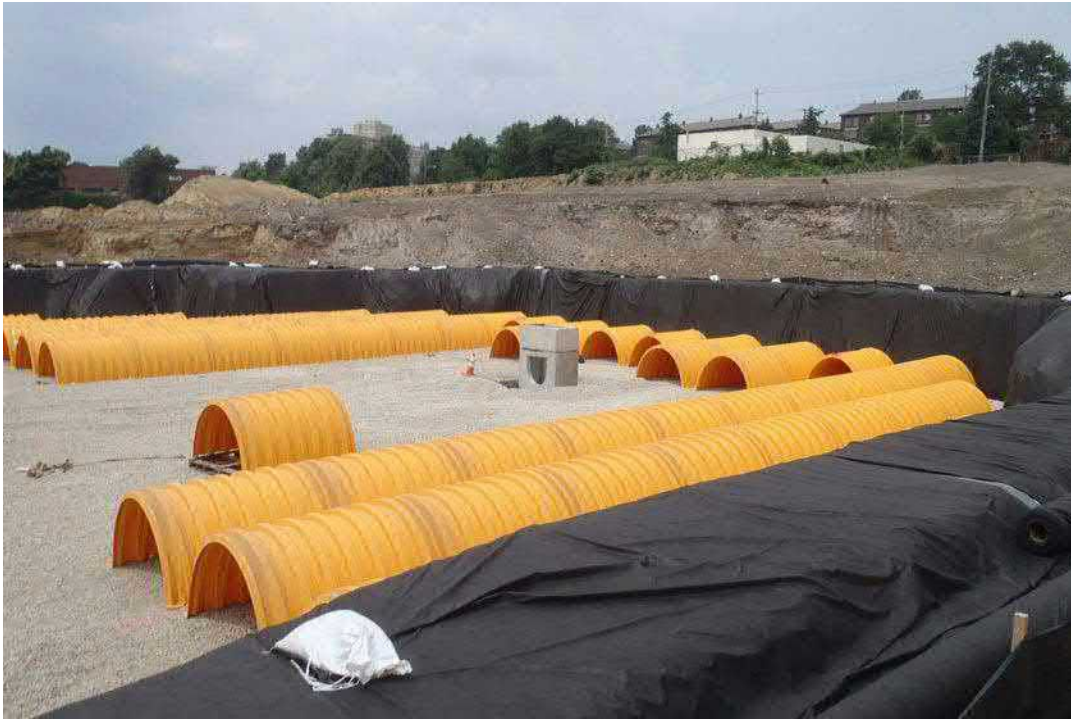
Figure 6.6.1: Subsurface Detention Storage Under Construction (photo c/o The Philadelphia Water Department, Stormwater Management Guidance Manual)
