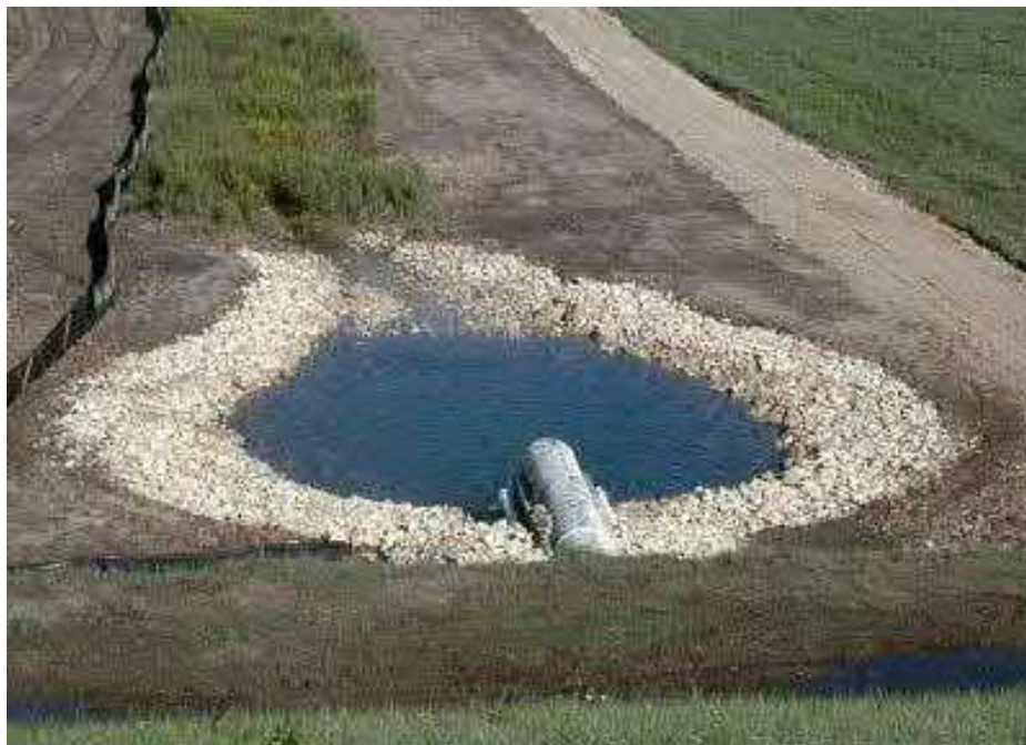
Plunge Pool (photo c/o PADEP Erosion and Sediment Pollution Control Program Manual)
