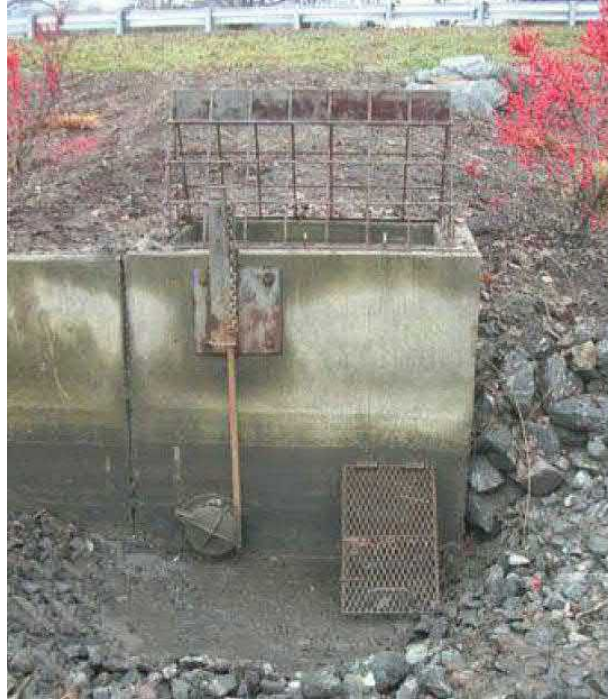
Figure 6.2.3: Lift-Type Sluice Gate (c/o NCDot-HSP-2010-01)
