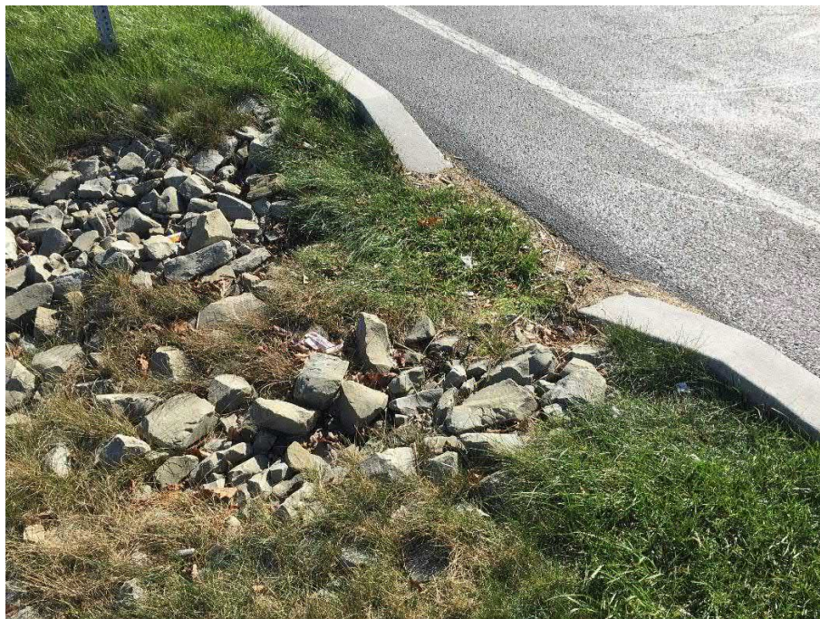
Figure 5.4.1: Inflow System- Curb Cut (photo c/o: PTC)
