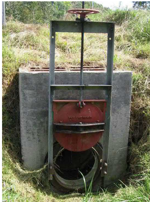
Figure 6.2.4: Open Screw-Type Sluice Gate (c/o NCDot-HSP-2010-01)
