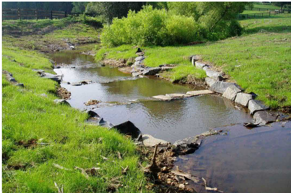
Stream Restoration- Cross Vane Structures
