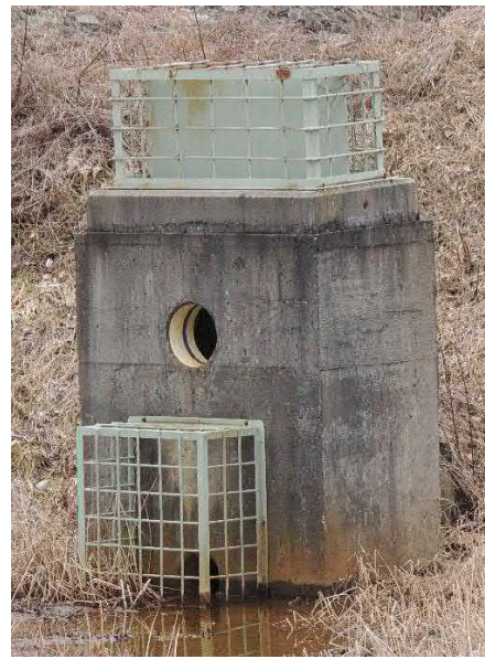
Circular orifices with trash rack on low flow orifice and top (photos c/o: PTC)
