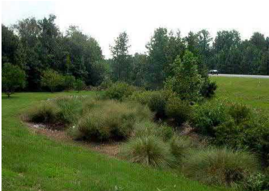
Figure 6.4.1: Bioretention
