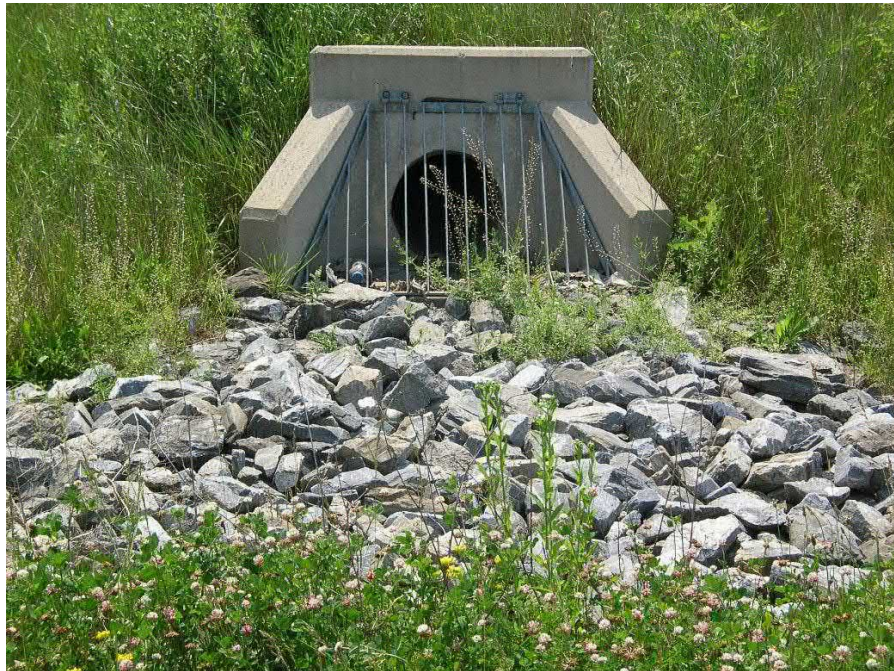
Endwall with Trash Rack (photo c/o: PennDOT)
