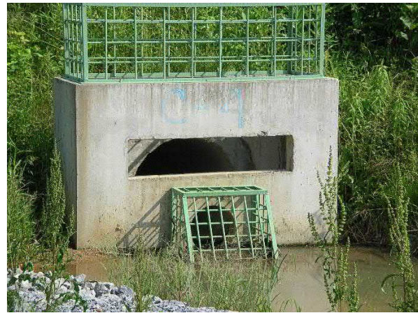
Rectangular weir & circular orifice with trash rack (photos c/o: PennDOT)
