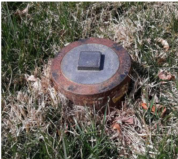
Metal Cleanout/Observation Well Lid
