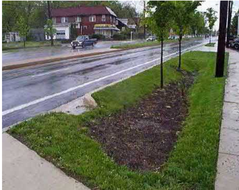
Figure 6.5.1: Subsurface Infiltration Trench (photo c/o: PennDOT)
