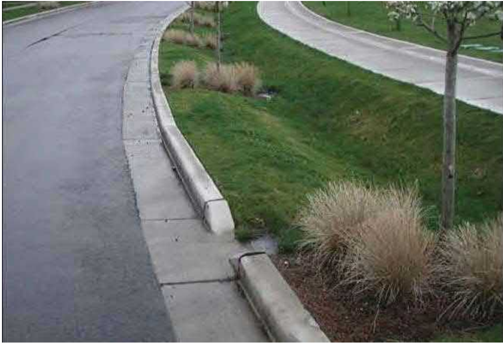
Figure 6.11.1: Vegetated Swale (VSW) (photo c/o Philadelphia Water Department, Stormwater Retrofit Guidance Manual)
