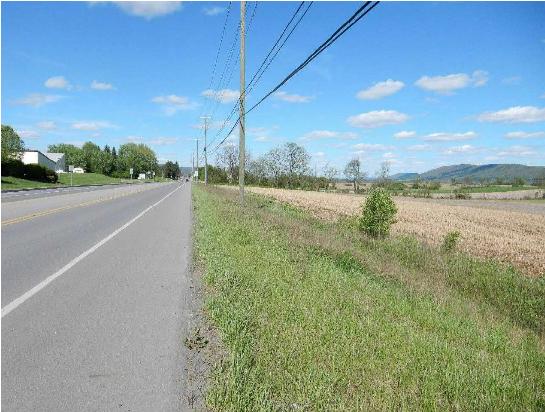
Figure 6.9.1: Vegetated Filter Strip (VFS) (photo c/o: PennDOT)
