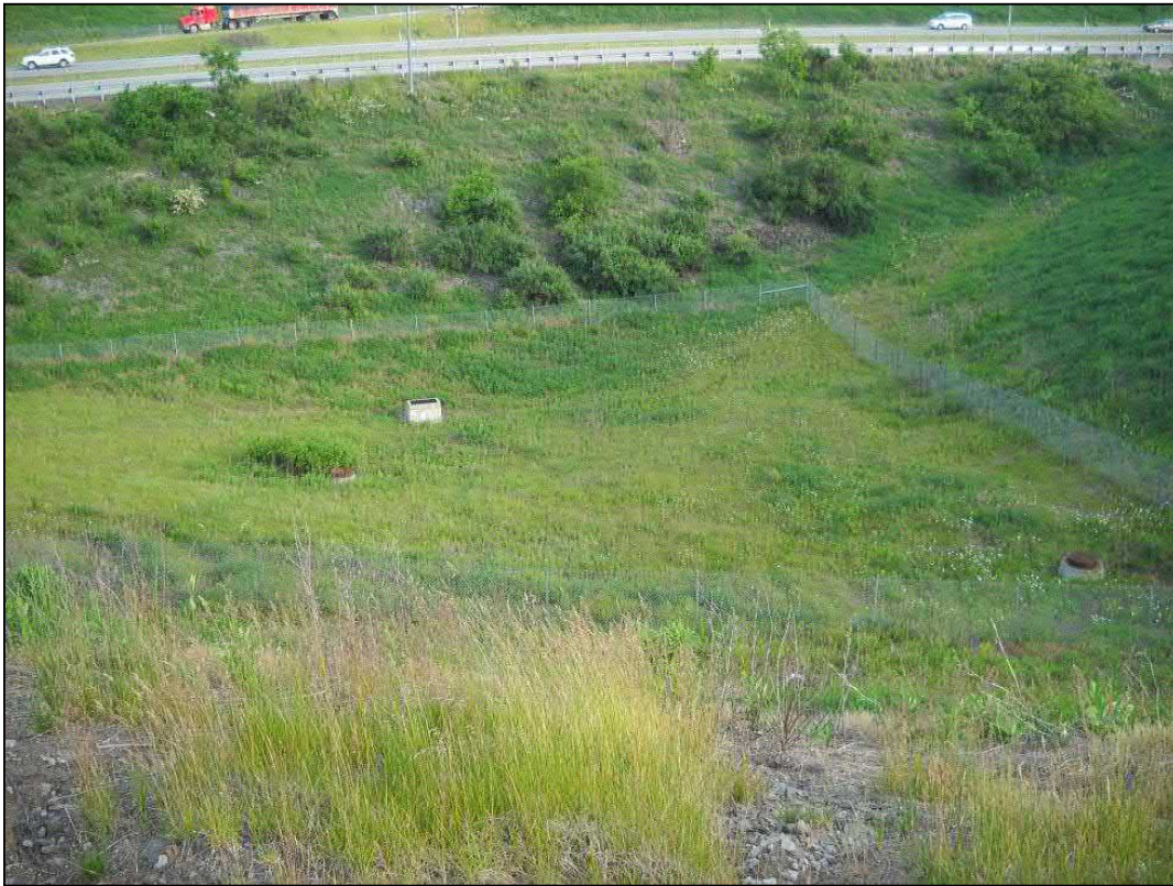
Figure 6.1.1: Dry Extended Detention Basin (photo c/o: PennDOT)
