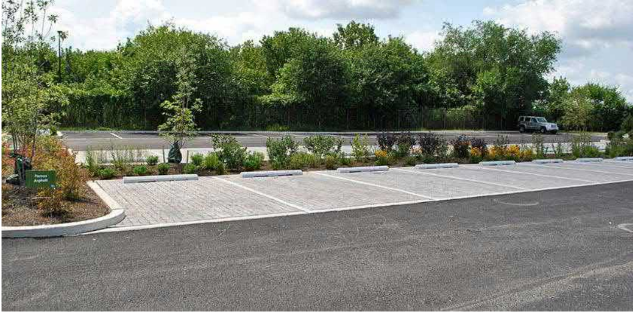
Figure 6.15.1: Pervious Pavement Pavers (PPP) (photo c/o The Philadelphia Water Department, Stormwater Management Guidance Manual)
