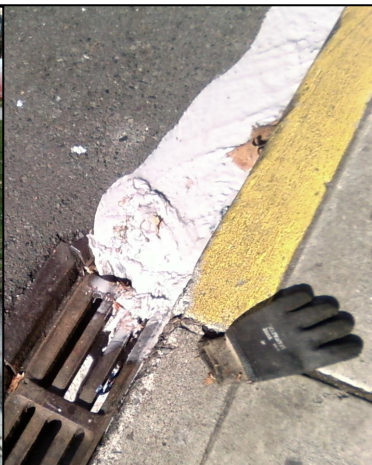
Paint/Plaster/Concrete Washout
