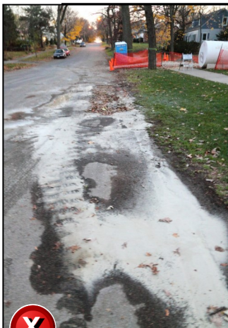
Paint/Plaster/Concrete Washout
