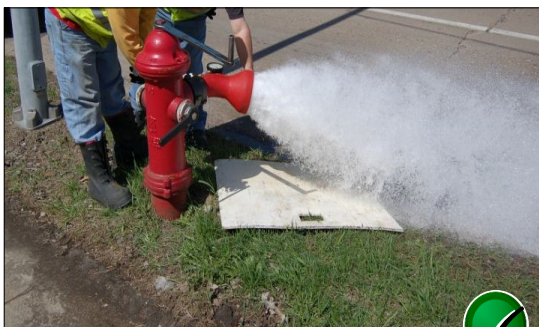
Water Line Flushing
