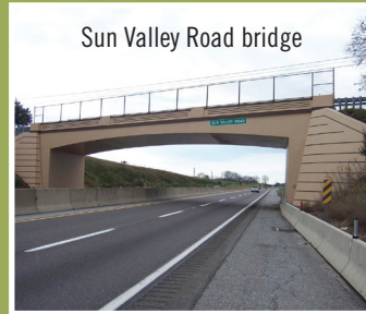
Reinforced Concrete Rigid Frame – 38
