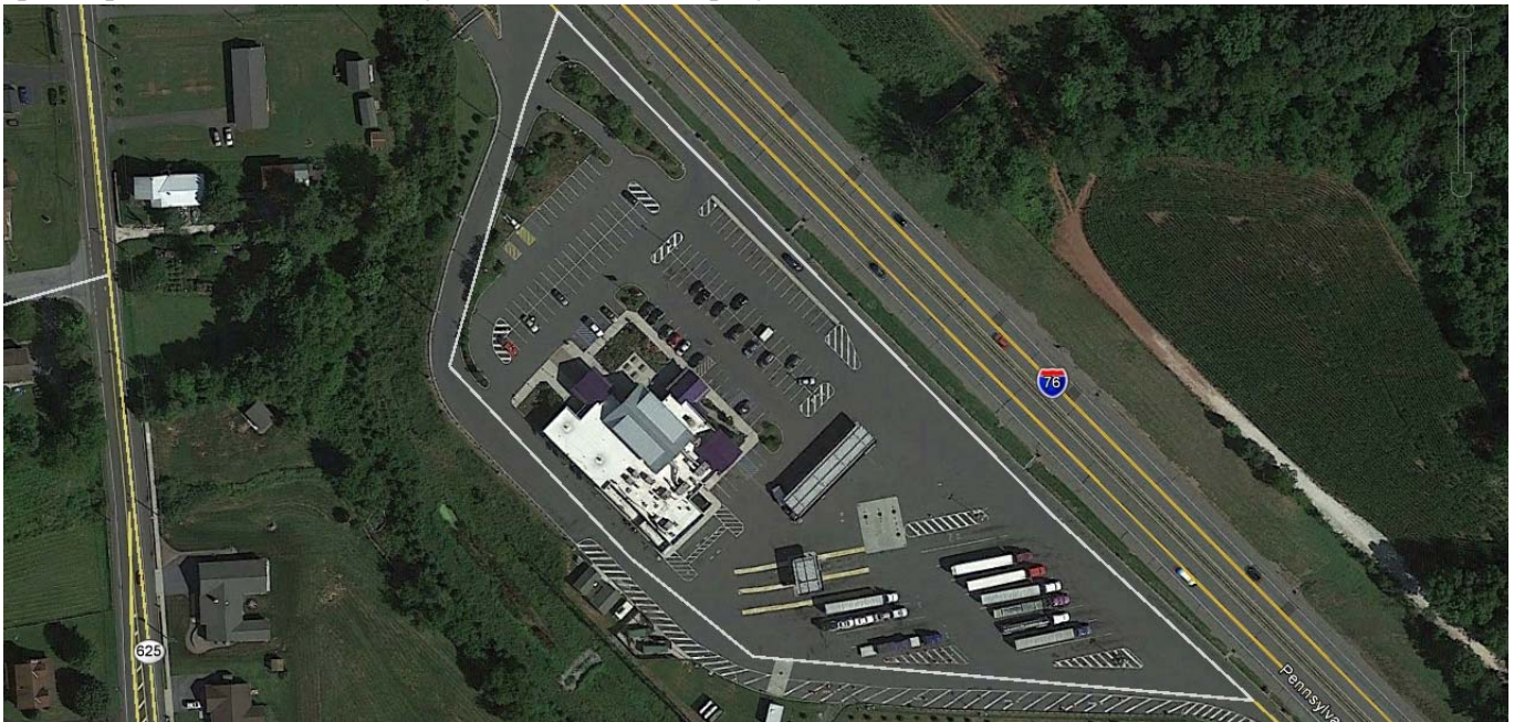
Figure 9: Bowmansville Service Plaza - Milepost 289.9 Eastbound
